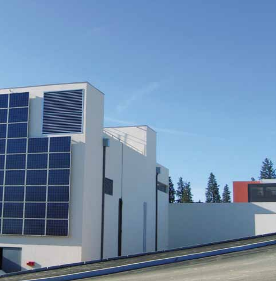
The energy pole at the Alès General Hospital, France.
