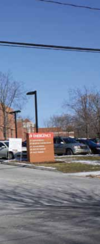
The new Milford Hospital in Connecticut, USA, is brimming with sustainable healthcare initiatives.
