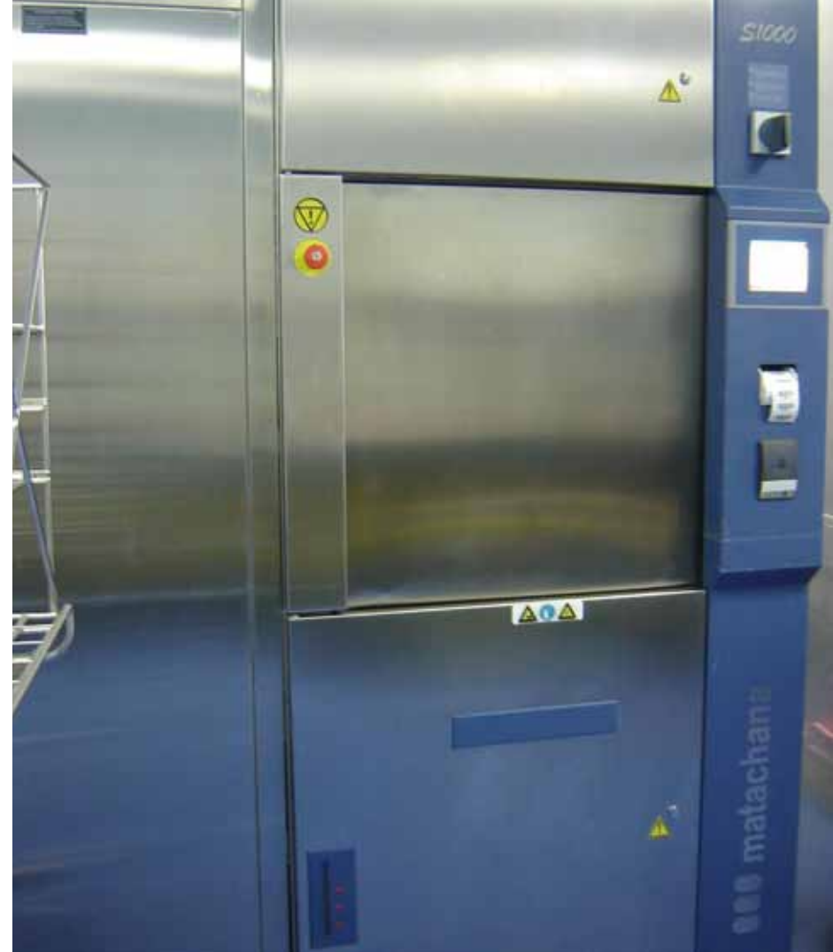
The autoclave at the Pasteur Clinic in Royan, France, uses between 20 and 25 liters of water instead of 250 liters.
