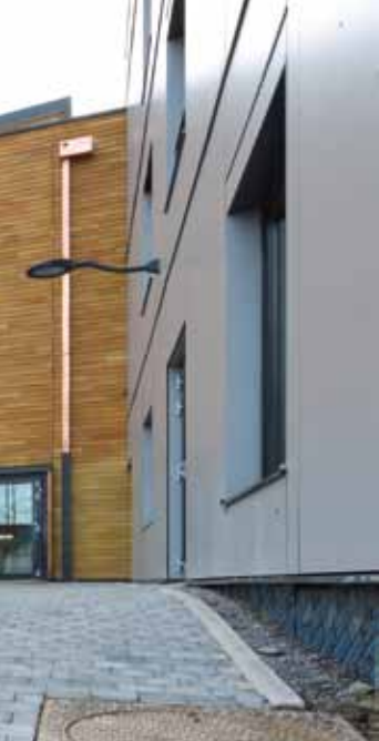
The Saint-Roch Clinic, France, gymnasium uses slabs made of the local wood, Locust.
